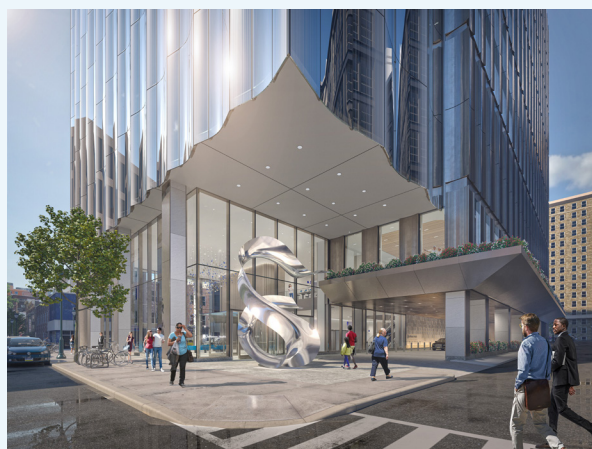
As the third-tallest building east of Broad Street, the Specialty Care Pavilion at 1101 Chestnut Street will transform the Center City skyline.
