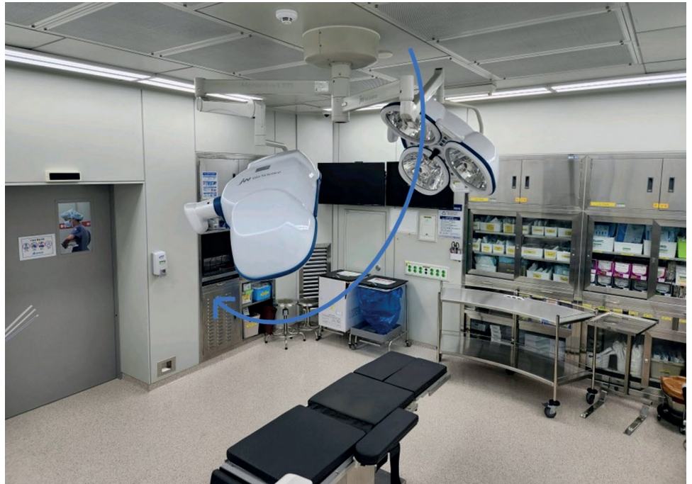
Fig. 2. All objects along the stream of air flow can shed particulates. The astral lamp, its lever and handle should be kept clean.
