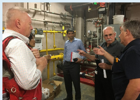
Jefferson Frankford Hospital Jim Creighton, AECOM, Damee Choi, AECOM, Alpeh Dharia, AECOM, Randy Haines, Director of Energy Management, Tim Mang, Supervisor
