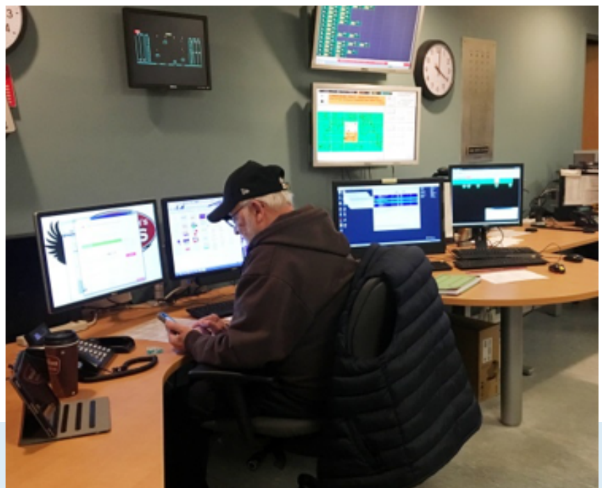
Tom McHugh at work in the Facilities Control Room.
