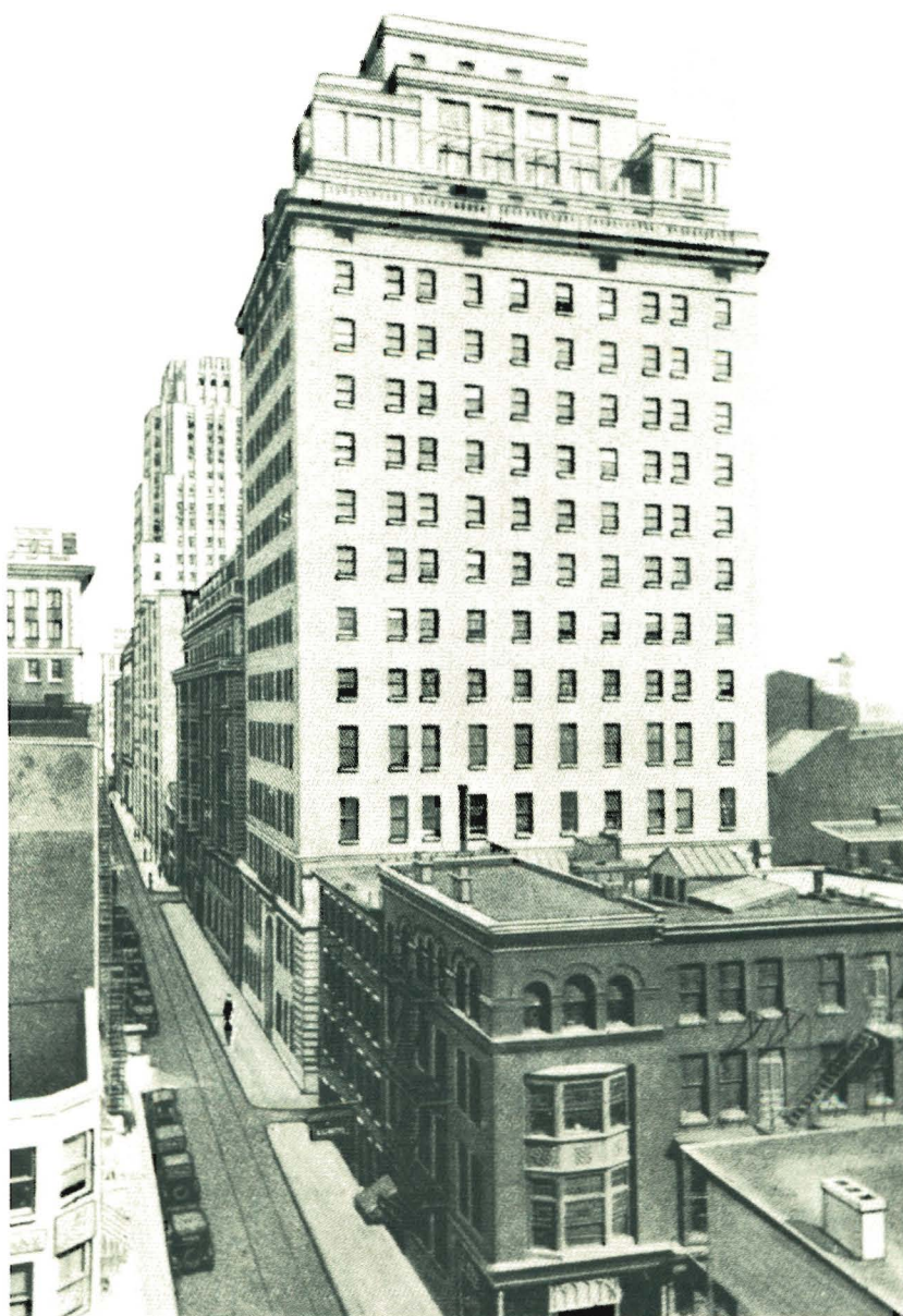
Fig. 230. Thompson Annex, dedicated October 30, 1924, at site of original 1877 Hospital.
