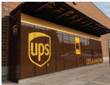
UPS Access Point
