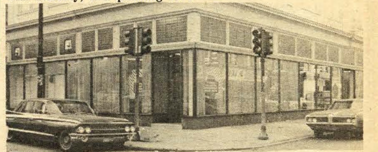
The present health center is located at the corner of ninth and South Street. (Photo - MCL.)
