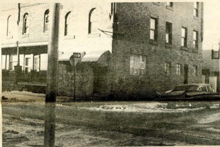
The clinic building at Gray's Ferry!
